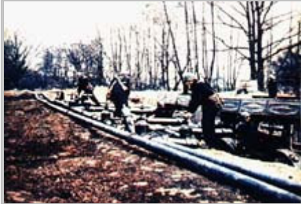
"The NVA were laying a Soviet-made tactical fuel pipeline, like this one, near RT Kansas' hilltop, the first ever extended into South Vietnam. It would be of strategic value a few months later during the Easter 1972 Offensive." (Def. Intell. Agency)
